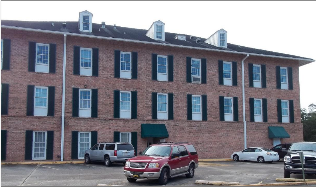
Figure 4-3: New Iberia City Hall hardened with functional hurricane shutters
